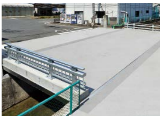
Road bridge employing aluminum floor slabs
