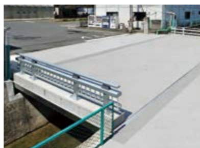
Road bridge employing aluminum floor slabs
