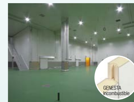
GENESTA Incombustible in use at a food processing plant
