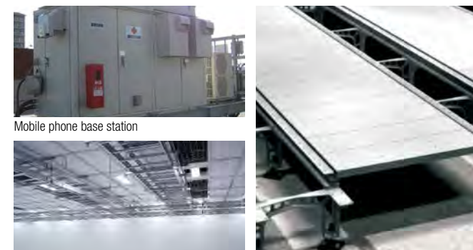
Nikkei server room and systems | Aluminum double flooring
