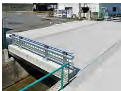
Road bridge employing aluminum floor slabs
