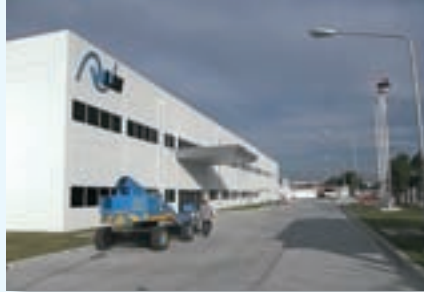
Exterior of new plant
