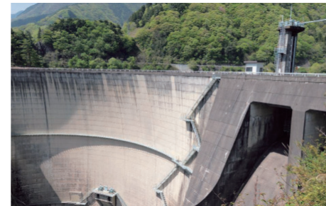
Overall view of the Amehata Dam
