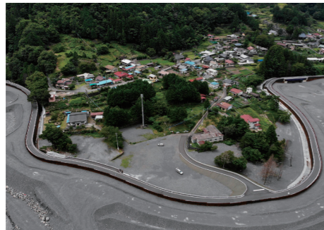
Embankment upstream of the Amehata Dam (taken in August 2021)
