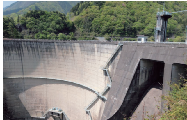
Overall view of the Amehata Dam
