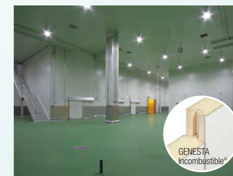
GENESTA Incombustible® in use at a food processing plant
