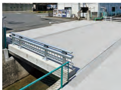
Road bridge employing aluminum floor slabs
