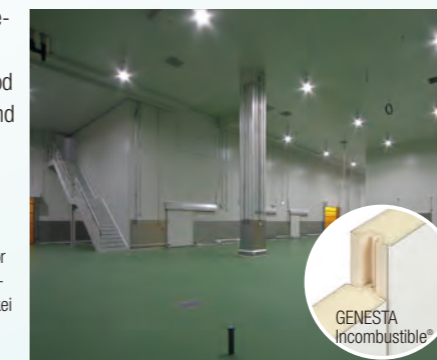
GENESTA Incombustible® in use at a food processing plant
